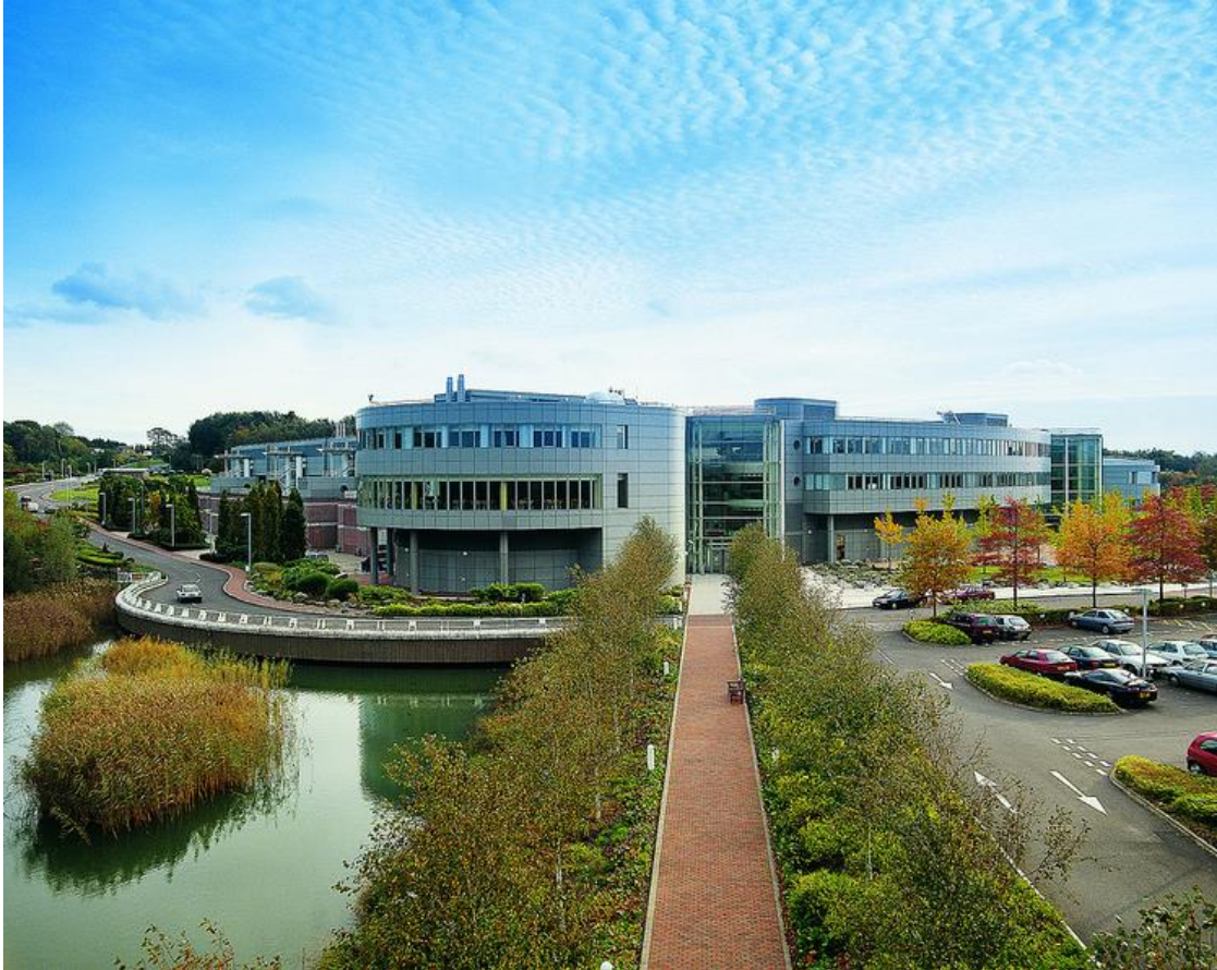
NATS: Control Centre at Swanwick. Source: NATS Press Office.
