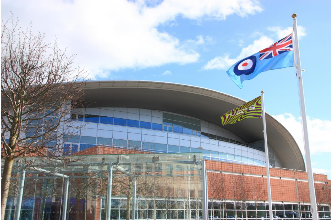
NATS Centre at Prestwick. Source: NATS Press Office.
