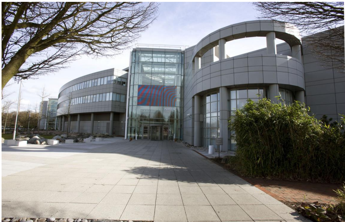
NATS Centre in Swanwick. Source: NATS Press Office.
